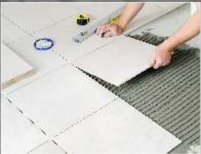
The tiles are placed with spacers and adjusted accordingly.
