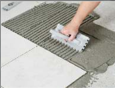
The tile adhesive is applied in a thin layer by means of a notched trowel.
